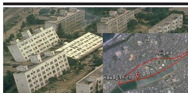
Figure 4. The effects of the 1964 earthquake in Niigata (Japan). The buildings were located in Kawagishi-cho, an area reclaimed from the river (red line). Wikipedia and Google Earth.
