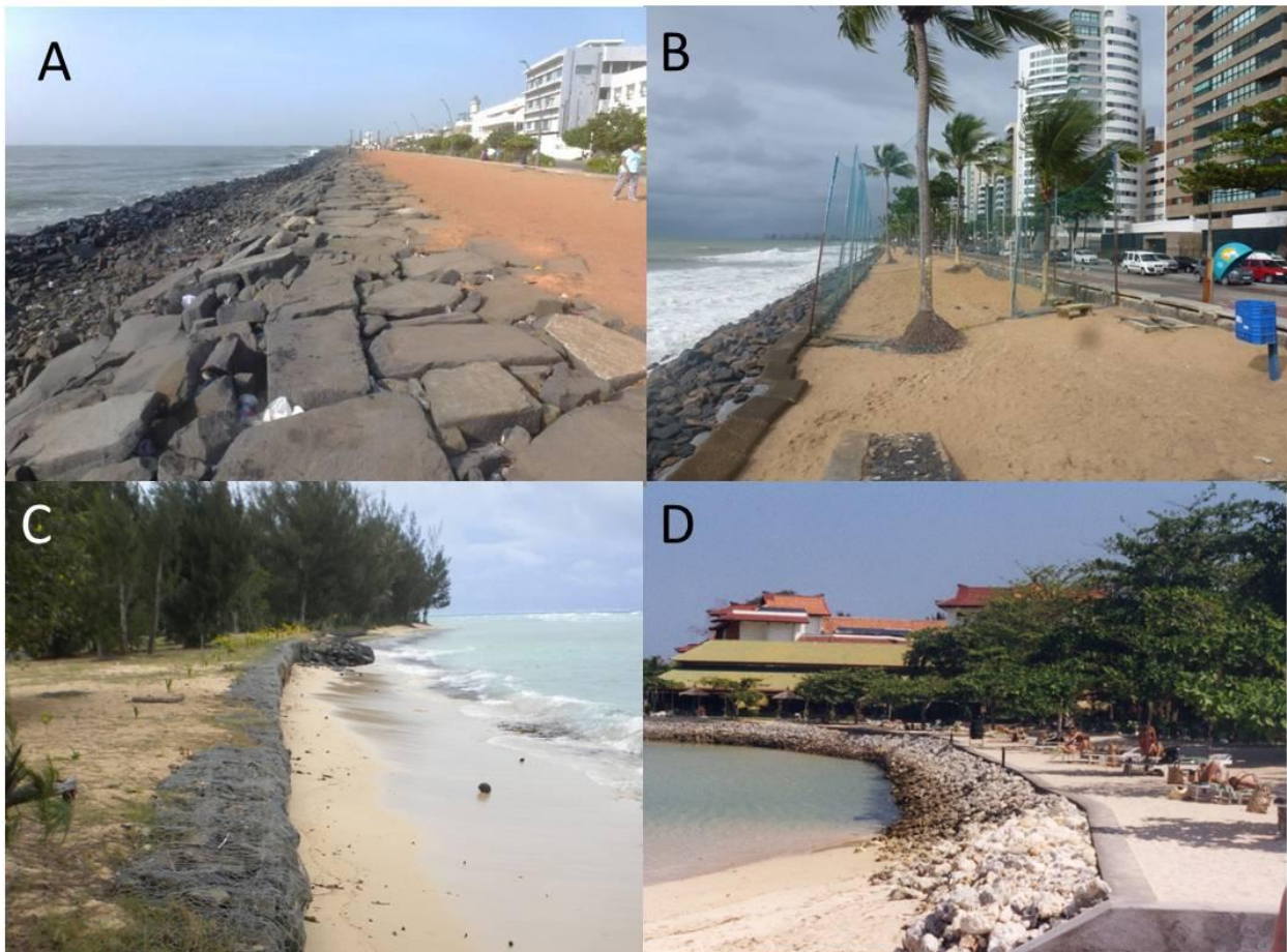
Figure 3. Various types of seawalls destroy beaches and cause loss of recreational potential as well as ecosystem functioning. A) The former beach at Pondicherry, India replaced by a seawall. B) The former beach at Recife, Brazil, replaced by a seawall. Note the beach volleyball pitch constructed in a sandpit on top of the wall. C) Gabion baskets at the rear of a beach in Tubuai, French Polynesia. D) The tourist resort of Nusa Dua, Bali, Indonesia where beaches have been replaced by concrete structures.
