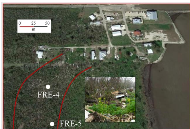
Figure 2. Frenier coring site. Red lines mark the approximate boundaries of a fairly narrow debris field resulting from Hurricane Isaac. As the debris originated in the lakeside buildings, the location and orientation of the field indicate the primary direction (from the northeast) of wind and waves at the time of maximum impact. Cores FRE4 and FRE5 were sited within the debris field.
