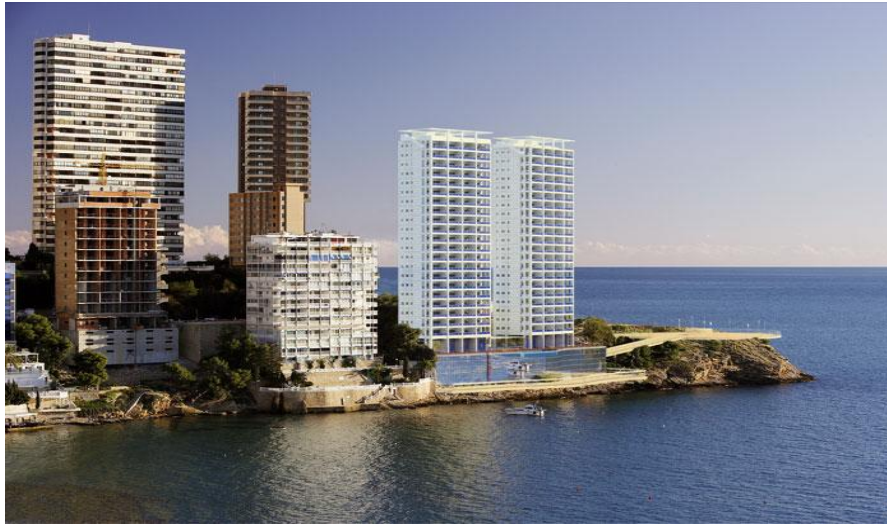
Figure 1. High rise buildings in the coastal environment (Benidorm, Spain) (M.A.R.M., 2013)
