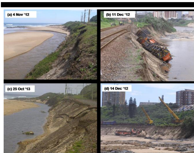
Figure 8: (a) Southward view of Amanzimtoti lagoon outlet showing slippage of the embankment on 4 November 2012. Note how close the slippage is occurring to the railway line and mast poles; (b) northward view of derailed locomotives and railway carriage on 11 December 2012; (d) inland (WSW) view of collapsed embankment and cranes to remove locomotives – note the lack of vegetation on the embankment compared to (a). Figure (c) is a southward view of the Amanzimtoti lagoon outlet on 25 October 2013, similar to that in (a), showing the outlet extended further south undermining the dune and ramp on which the white vehicle in the distance is parked. Note the absence of vegetation compared to Figure (a) as a result of continued slope failure.
