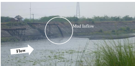
Figure 5. The mud inflow situation at the 26 K.P. on November 13, 2013. The picture was taken from the right side levee of the Porong River by the authors.
