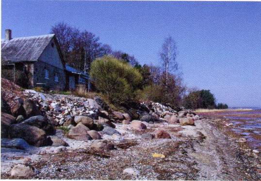
■ Figure 4.18 Boulder revetment at Valgalciems (western coast of the Gulf of Riga)
