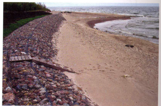
■ Figure 4.20 Liepāja wastewater treatment plant revetment
