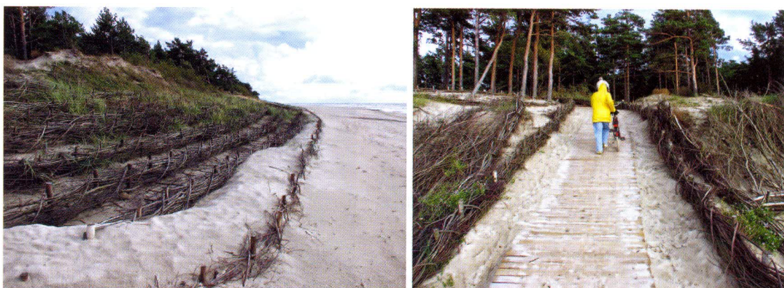
■ Figure 4.28 Foredune maintenance by elementary measures near Palanga
