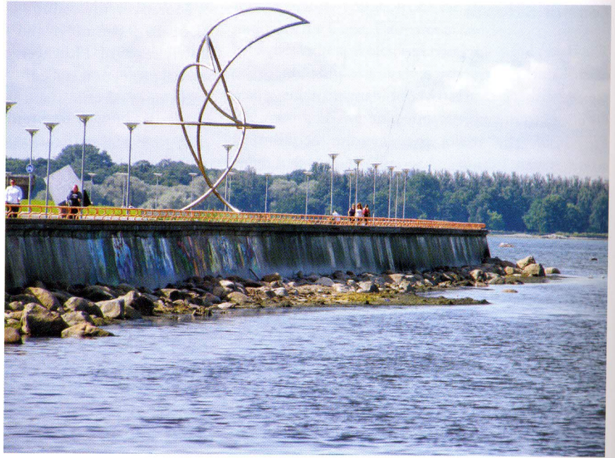
■ Figure 4.8 Seawall protecting Pirita roadway in Tallin Bay
